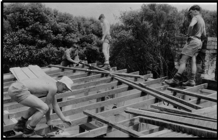
Re-roofing Ongaruanuku – November 1963 John Utting, George Brennon, Jim Frater.
