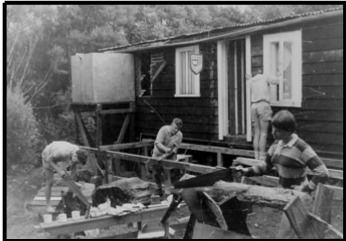
Building the new Verandah - April 1964
